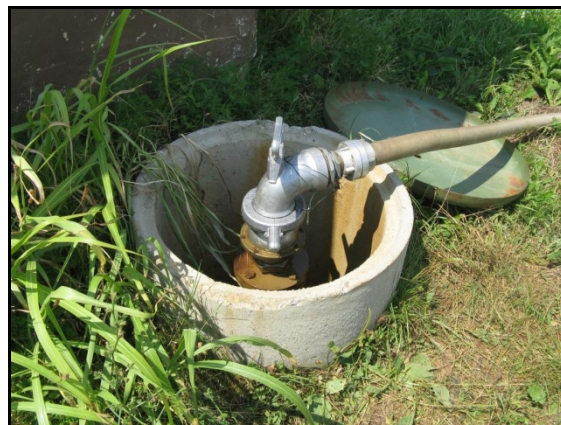
Slika 12: Hidrant namakalnega sistema za priključitev namakalne opreme (terciarnega voda) Figure 12: Hydrant on irrigation system for the connection of irrigation equipment
