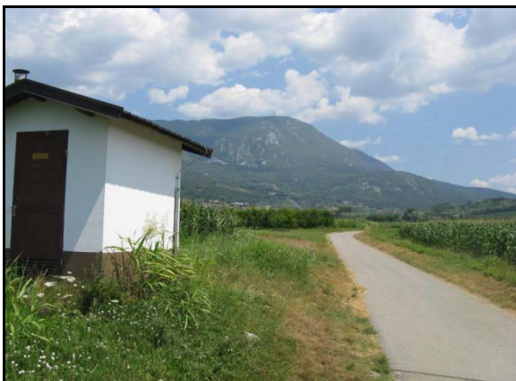
Slika 11: Objekt z odvzemnim/sekcijskim jaškom Figure 11: The building with an extraction/section shaft
