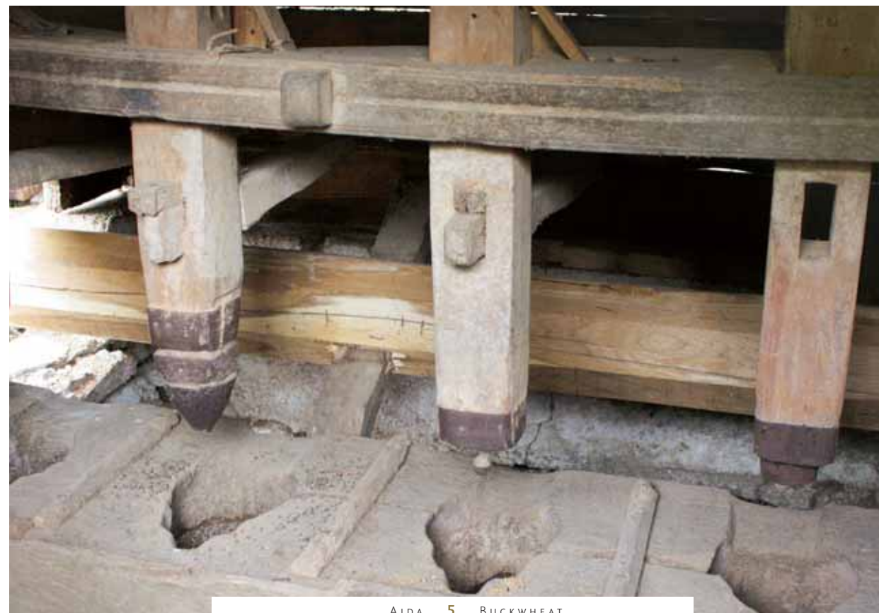
Stope na vodni pogon / Water-driven buckwheat dehusking device
